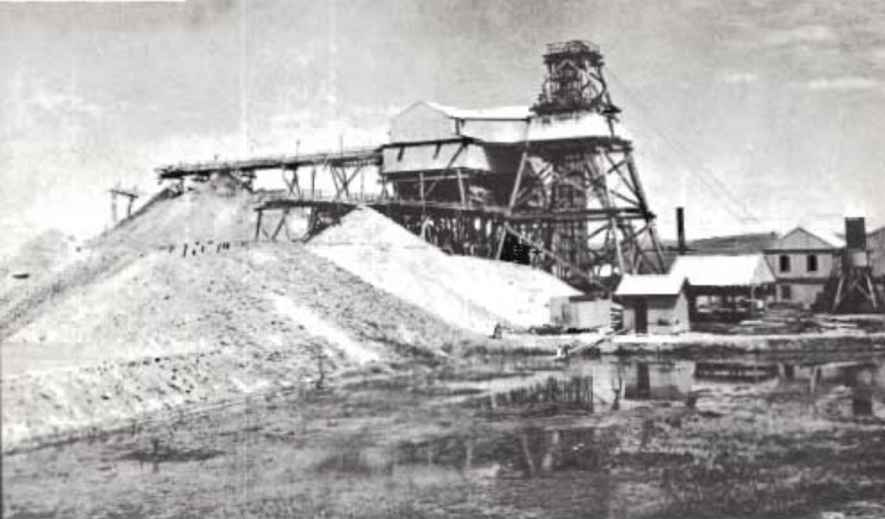
Poppet head and tailings of the Talbot alluvial mine, c. 1930s.
