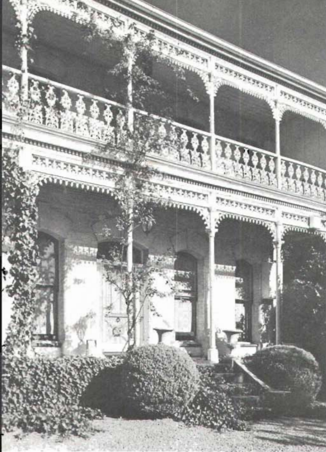
Ornamental ironwork on verandahs was a feature of many buildings from about 1860. Dr E. Graeme Robertson
