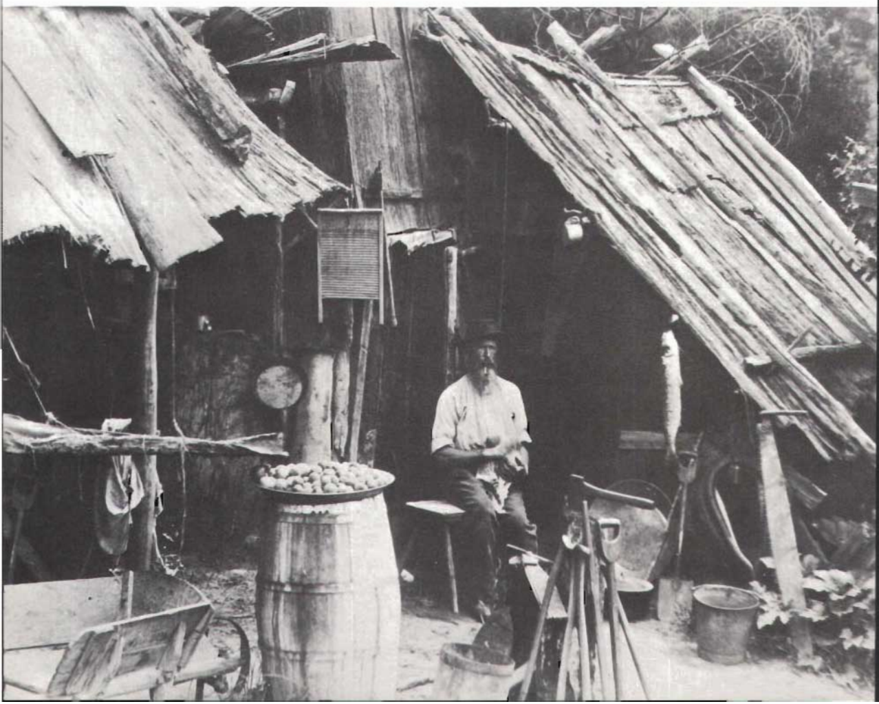
Selector's hut built of logs, slabs, and bark (but without nails) in east Gippsland.
