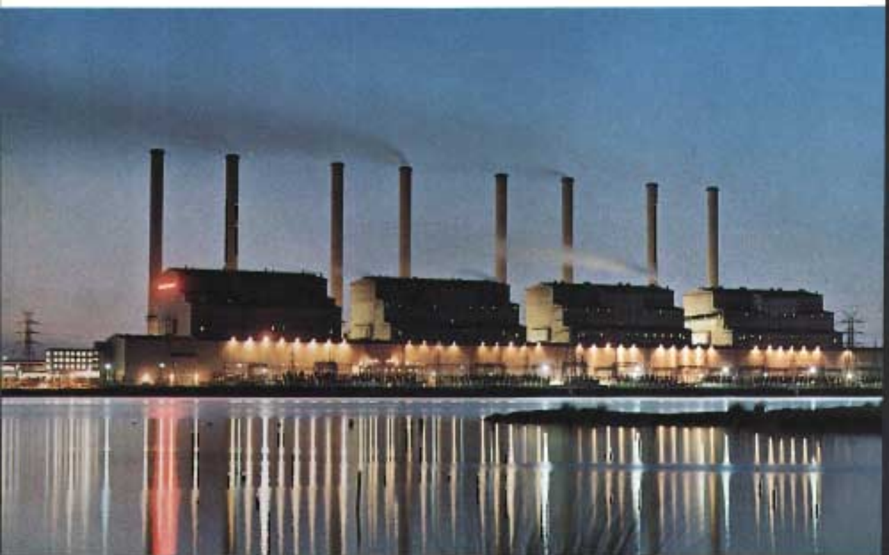
Hazelwood power station in the La Tröbe valley. State Electricity Commission
