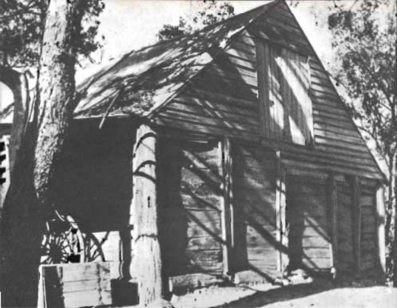
The roughly constructed slab shed has been a feature of many farms.
